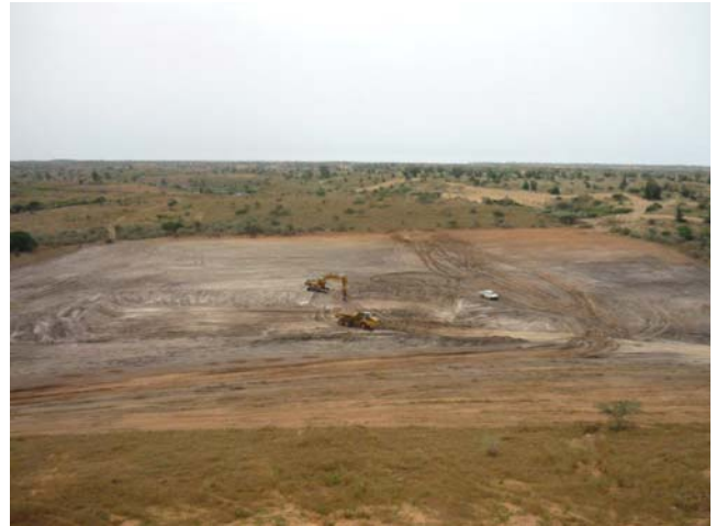
Preparation of the initial dredge site
