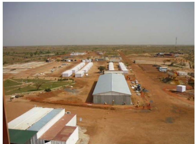
Construction camp taking shape
