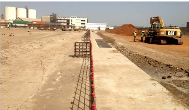
Civil works at Dakar port facility
