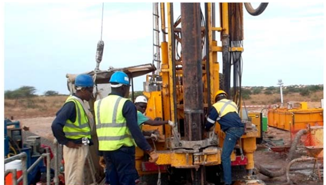
Drilling of deep water bores – 6 of 12 now complete
