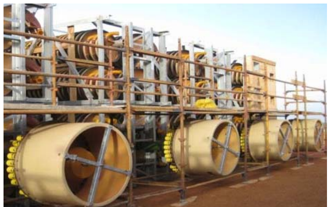
Spirals of WCP under assembly on-site
