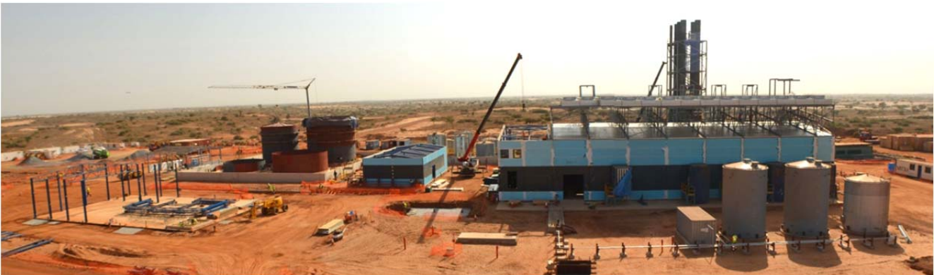
Power station construction
