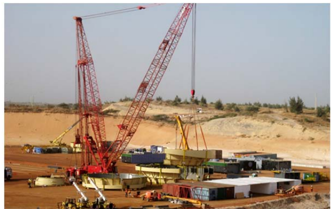
Surge bin of WCP being assembled on-site
