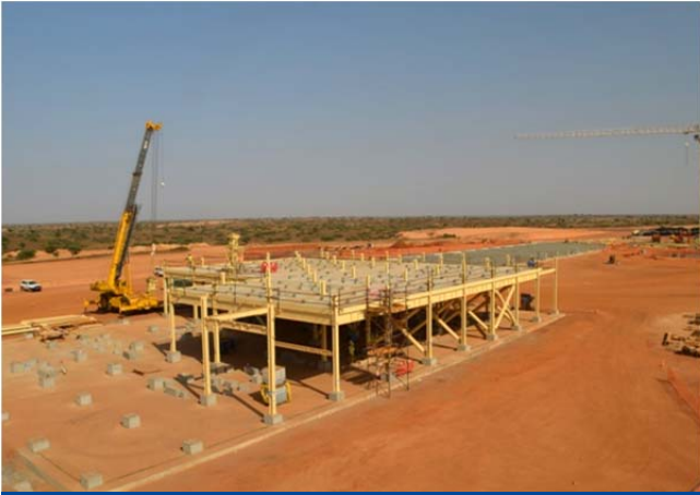
Wet mill at MSP taking shape
