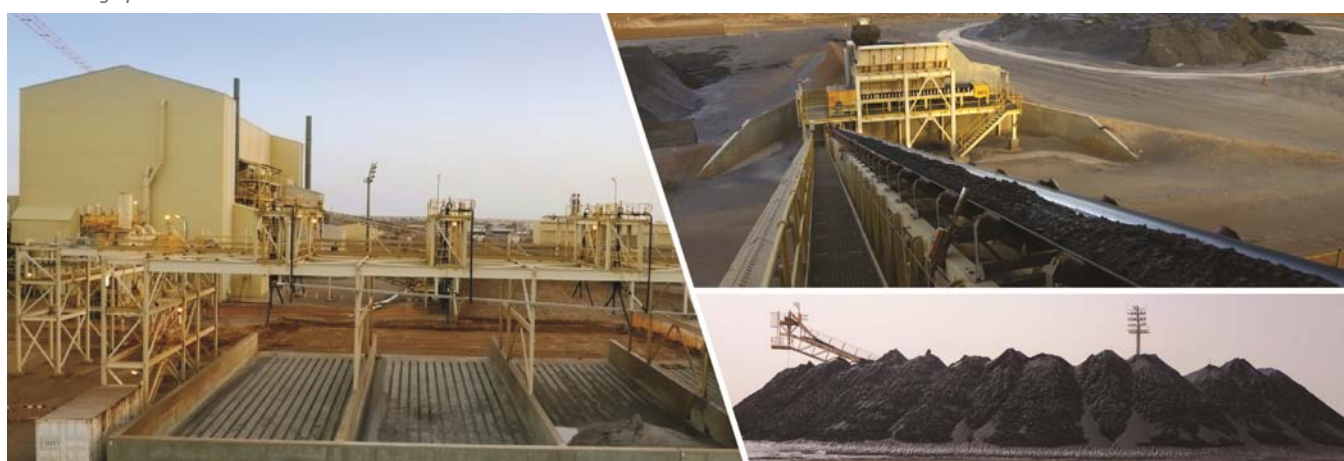
GCO Mineral Separation Plant
