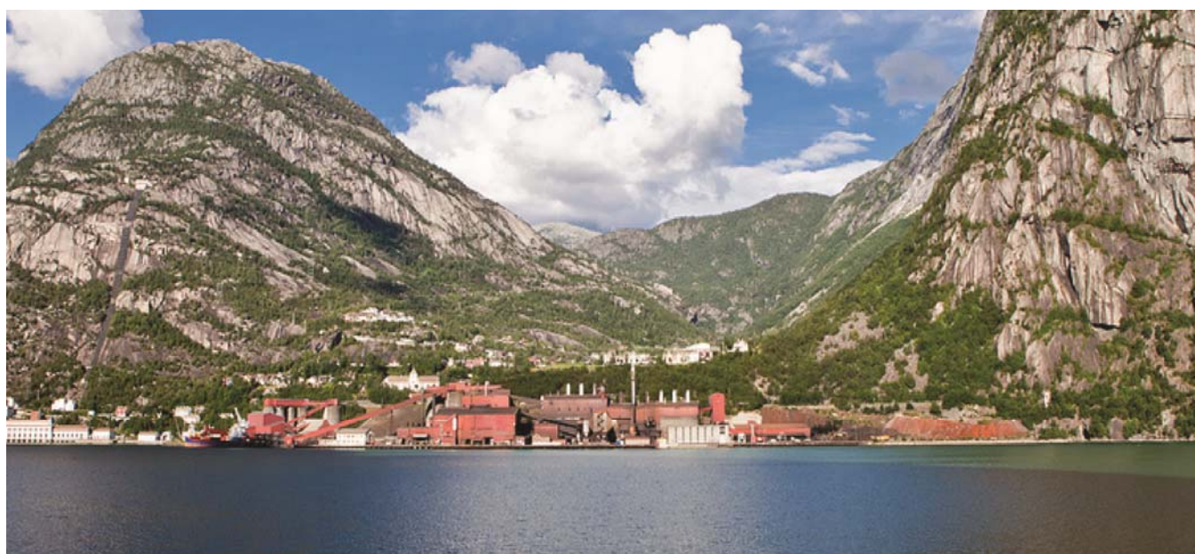
TiZir Titanium & Iron ilmenite upgrading facility, Norway
