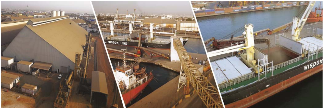
Storage and conveyor facilities at Dakar Port
